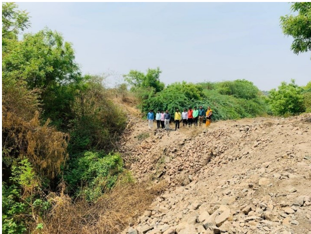
Rain water and waste water blocked and percolate in the soil which helps in increase in groundwater capacity behind the college building.
